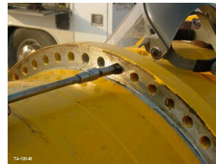
Cleaning paint and rust prior to torquing
