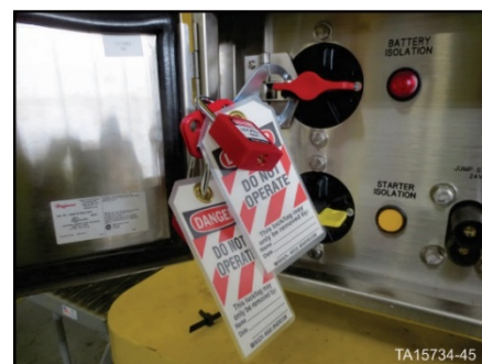
Battery isolation switch in OFF position with locks in place
